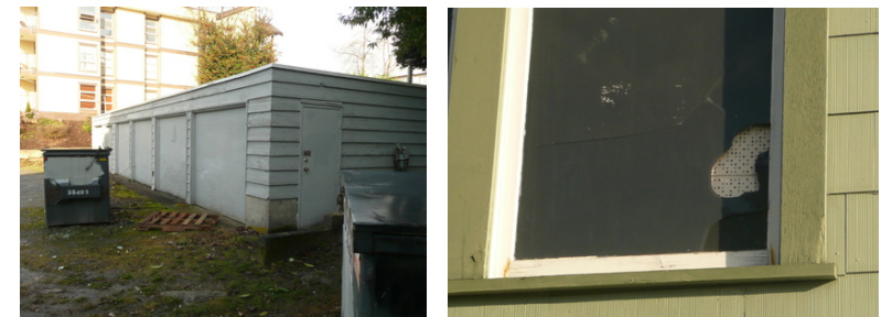
Deteriorated windows, deteriorated painted wood
